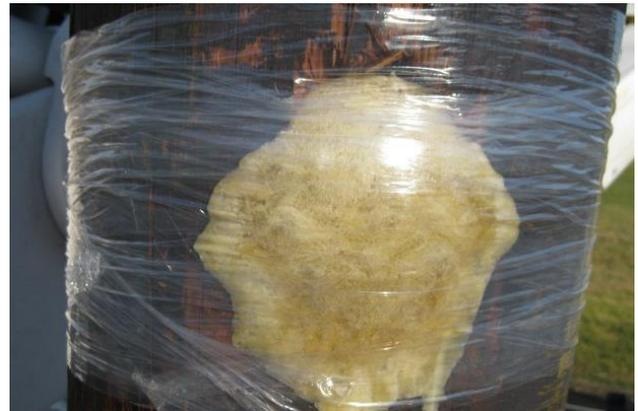
Woodpecker damage repaired with UPR™ Pole Repair
