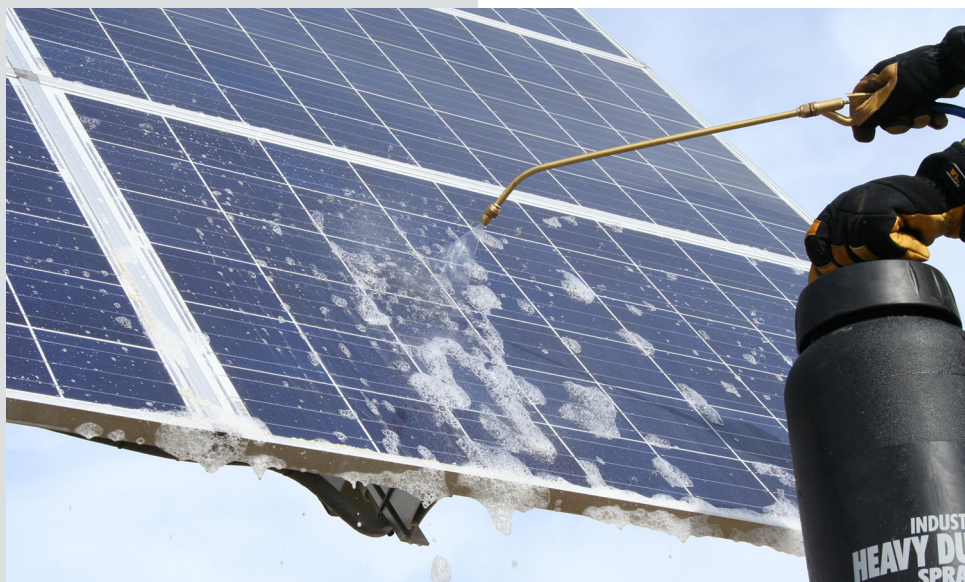
Polywater SPW sprayed onto panel surface
