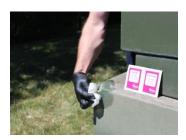
3. Match the fabric with the area to be repaired. Cut the fabric to overlap the damage by approximately 1" all the way around.
