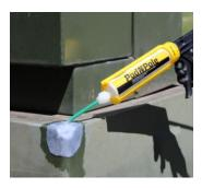
6. Generously apply additional Pad N Pole Repair to the top of the fabric and smooth with the brush until all of the fabric is saturated. Brush Pad N Pole Repair ½" past the edges of the fabric, smoothly feathering the Pad N Pole Repair and ensuring that the edges of the repair are well adhered to the pad, pole or enclosure. Pad N Pole Repair will cure in about 30 to 45 minutes and fully harden in 4 to 6 hours.
