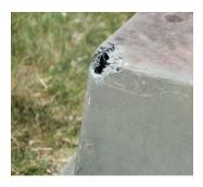
1. Examine the damage on the pad, pole or enclosure. If needed, dig out sod and soil to reveal at least 2" of undamaged surface around the defect.
