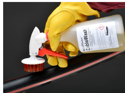
Cleaned cable jacket
